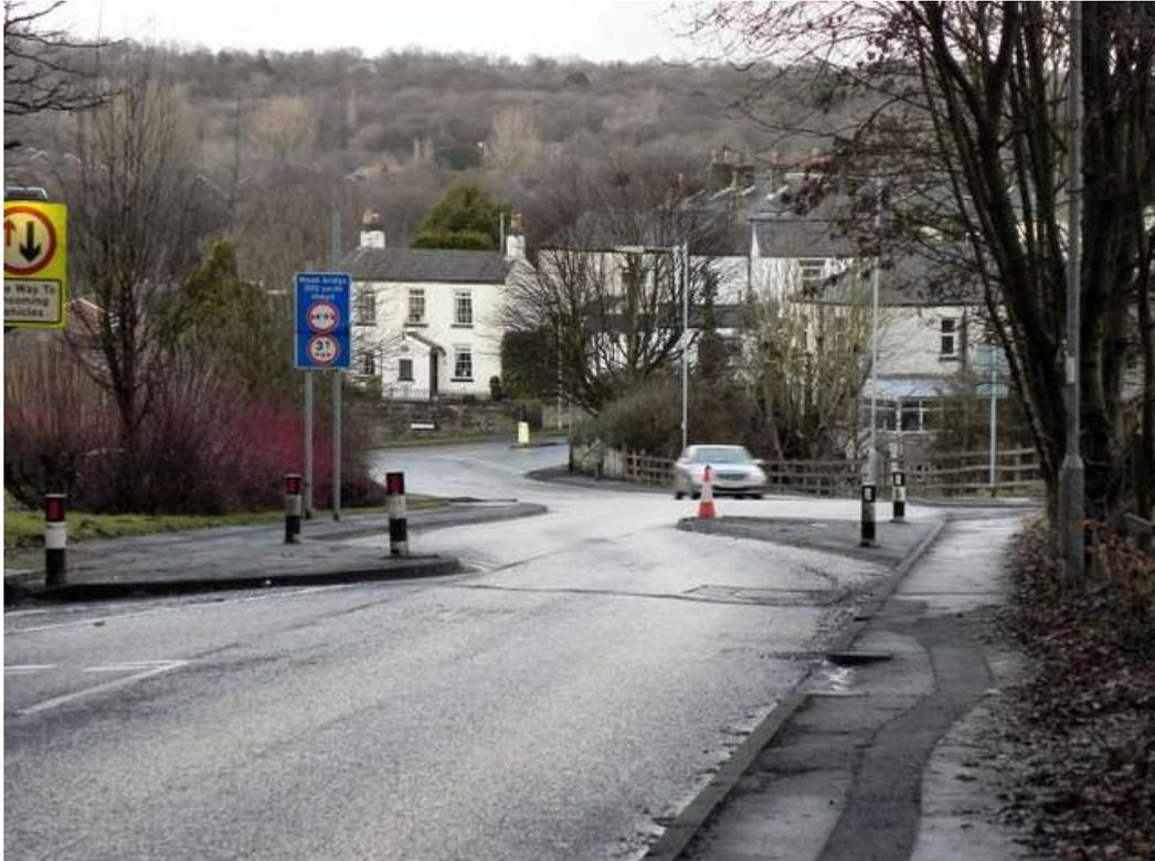
This particular version shows a sharp 'S' bend together with weight restriction and width restriction signs. It would not be difficult to construct at the junction with B5056 and would still allow passage of light vehicles and emergency crews. A device such as this would not, however, be as effective at the junction with Main St.
